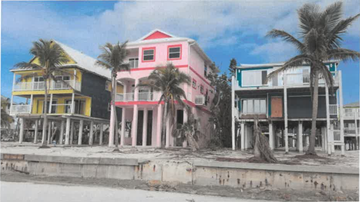
Figure 1: Three neighboring buildings with varying degrees of elevation and damage on Fort Myers Beach, Florida, after Hurricane Ian. The right-most building has the lowest elevation of the three and the most damage to the lower levels, whereas the middle building has the highest elevation and minimal damage to the lower levels.
